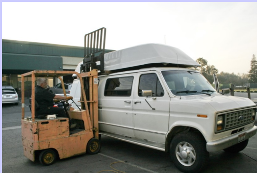
New roof goes on
