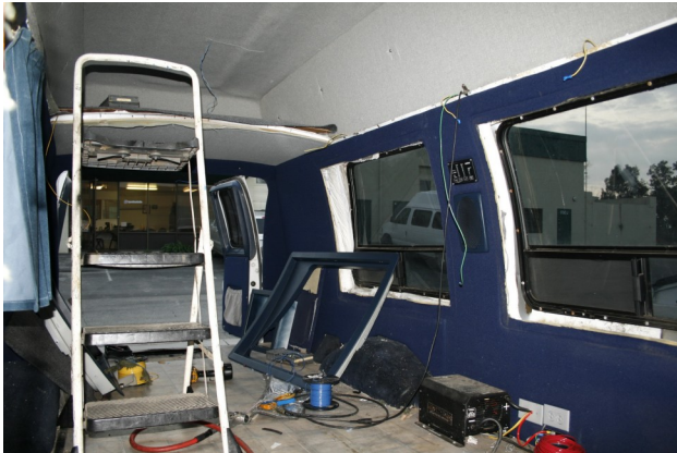
Torn apart with new roof and headliner .....to
