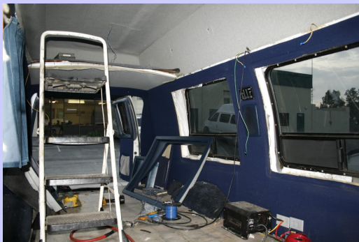
Interior work begins
